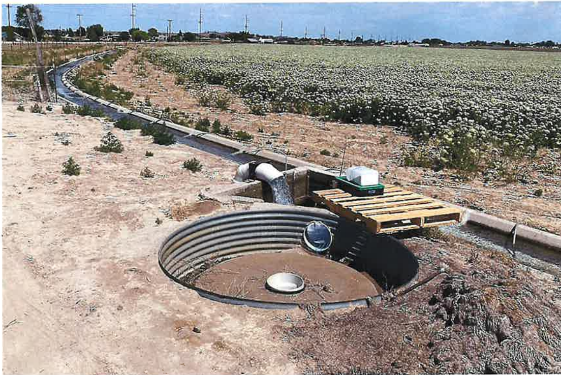
Discharge from well to concrete box looking north. Concrete ditch and field 2 in background. Delivery pipe from Mora Canal in foreground
