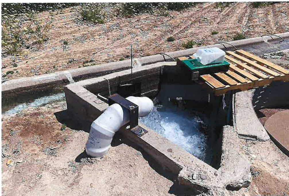
Discharge from well to concrete box looking east
