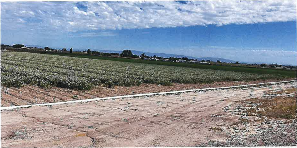
Gated pipe for irrigation of field 3
