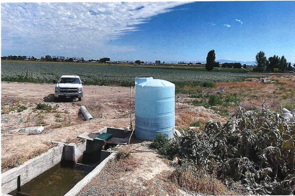
Delivery box and weir to field 23. Water can be pumped to this box from the pond (or from ditch) east of field 4.
