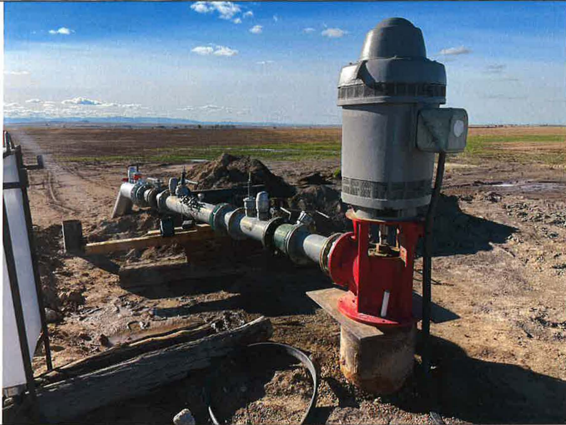
Point of Diversion
