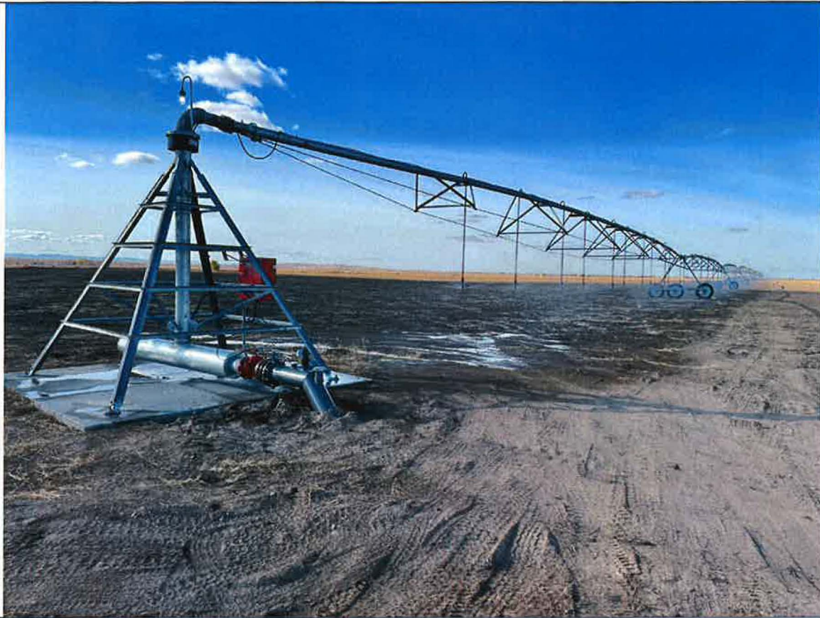
Pivot system and irrigation place of use.
