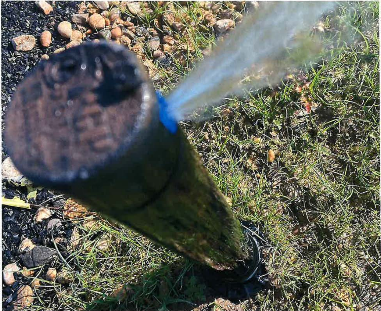
Figure 5: Hunter PGP Ultra with blue nozzle
