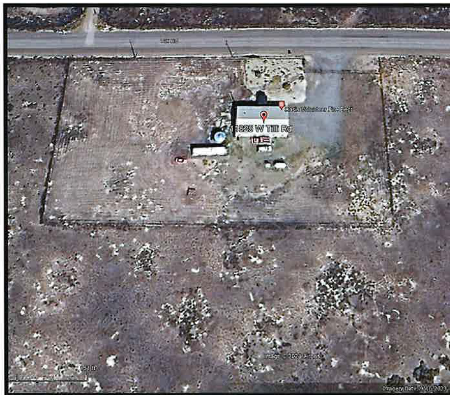
Figure 2- Google Earth 2023, image of the POU with the firehouse labeled with the street address. The round silver structure on the southwest corner of the building is the 2500-Gallon water tank.
