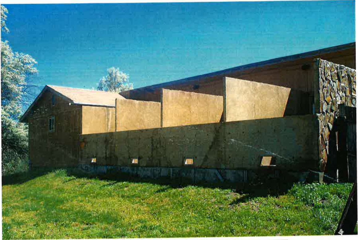
Un-finished Hot Baths At West End of Facility By J E Stanton 6-5-2002 Permit 47-7829
