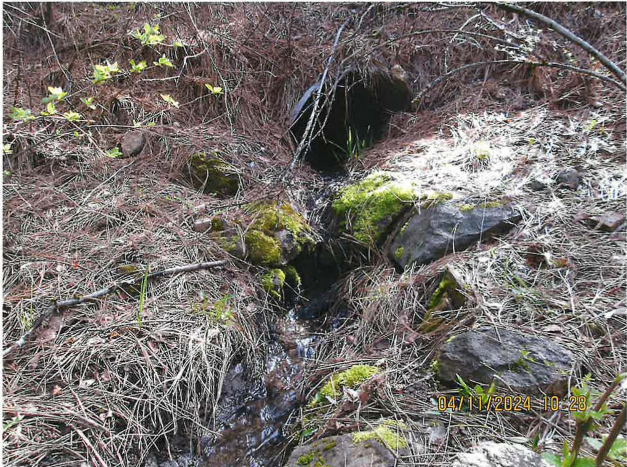
UNNAMED STREAM CULVERT
