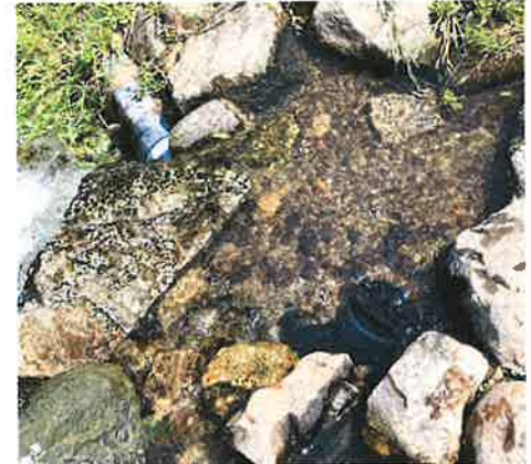
3" pipe with 1/4" screen cap at diversion intake point. Pipe is partially covered with rock at creek location and buried underground between creek and pond.
