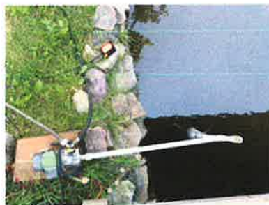
THE PUMP is located on the north-west side of the pond bridge. A mesh screen surrounds the intake pipe where it is located under water.
