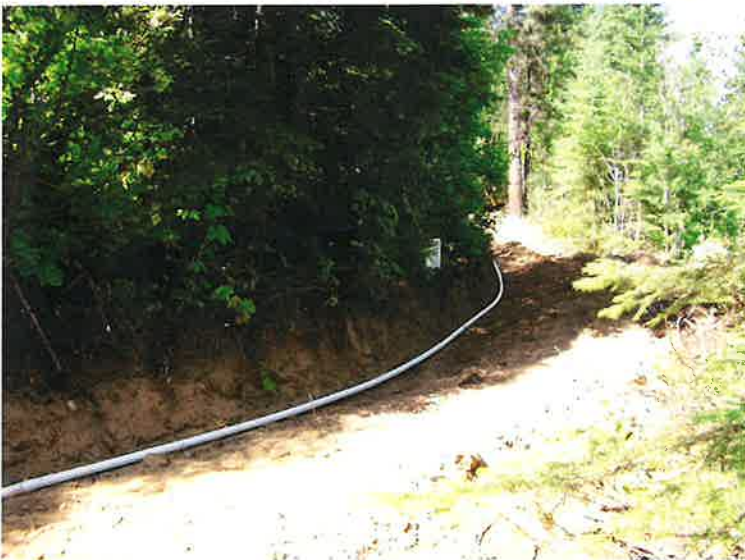
2" PVC water line instillation
