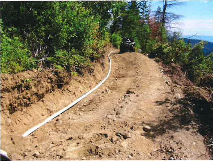
2" PVC water line instillation
