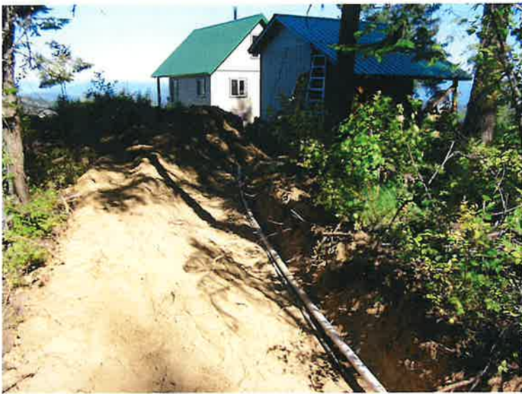
2" PVC water line instillation
