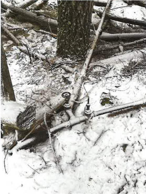
drainage valve and air purge to start flow
