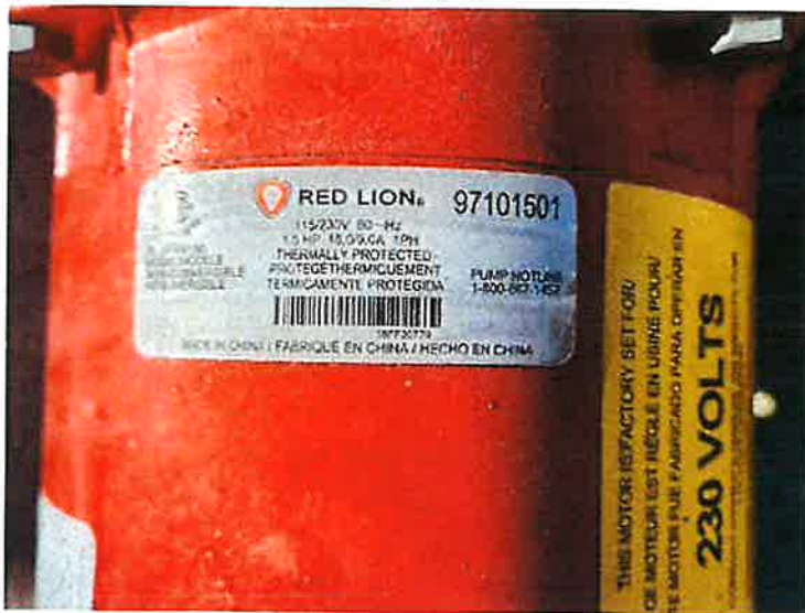
Figure 7. Pump used to pressurize sprinklers to irrigate 0.08 acre at the lower hatchery facility.
