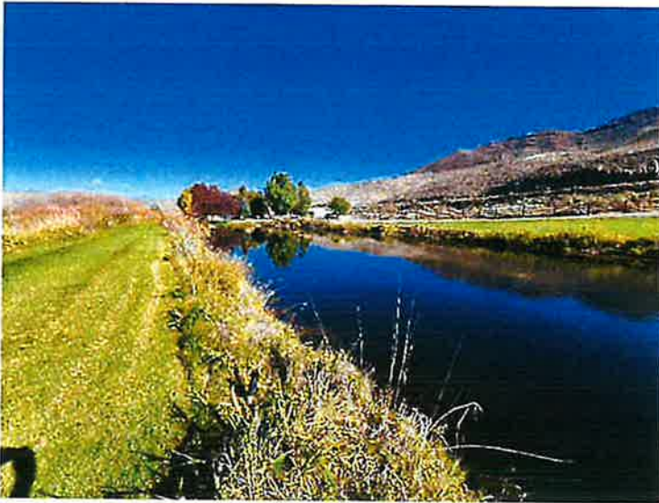
Figure 8. Water flowing downgradient of the fish screens prior to reaching holding ponds at the lower hatchery facility.
