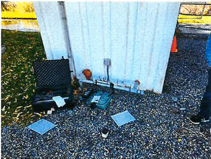
Figure 12. Straight length of pipe installed per 73-12269 permit condition number 5.
