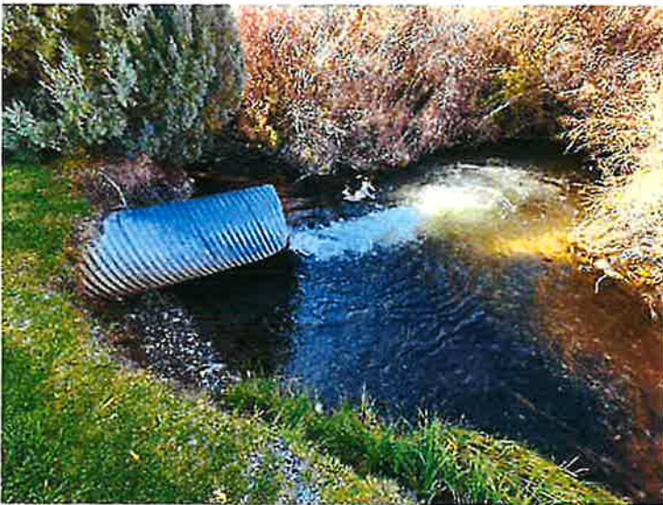
Figure 10. Water flowing from control gates bypass back to the Pahsimeroi river.
