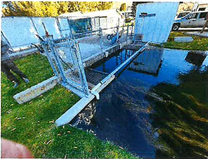
Figure 9. Water flowing from the unlined canal downgradient of the fish screens into the control gates of the holding ponds/structures at the lower hatchery facility. There is a bypass line in the foreground of the photo that conveys overflow water back to the Pahsimeroi river.
