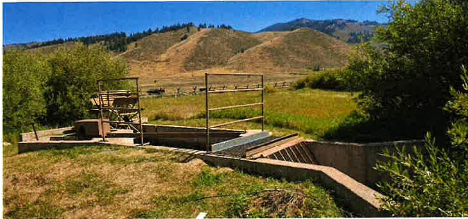
Figure 1: Fish Screen with bypass (notice t-handle on left side where bypass is located)
