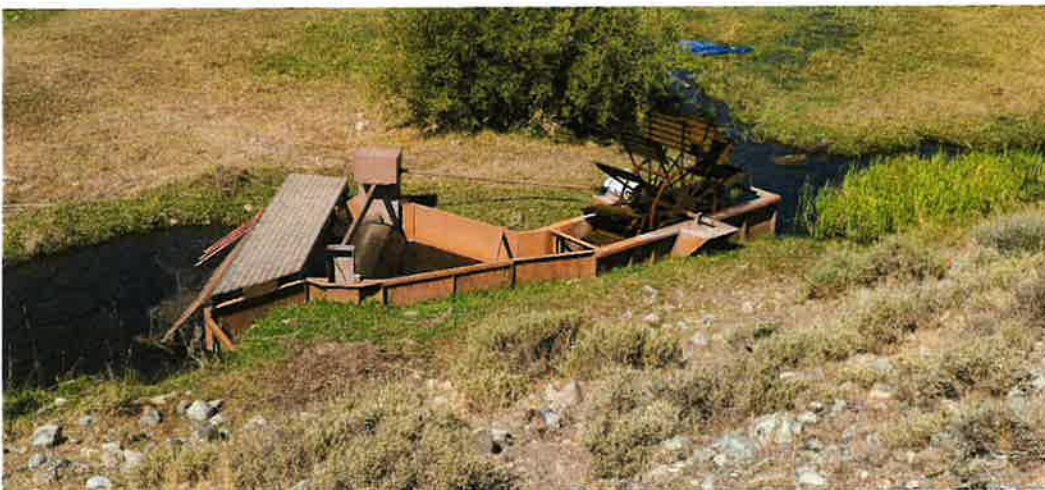
Figure 2: Fish Screen with bypass under far side of the walk screen (notice t-handle there)
