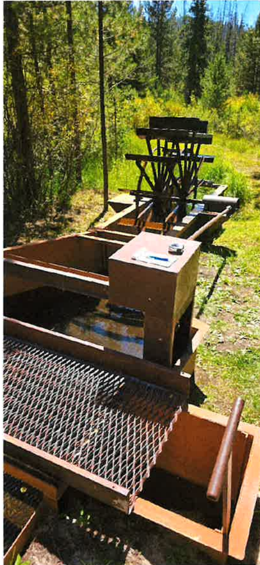
Figure 1: Fish Screen & Bypass (below handle in foreground)
