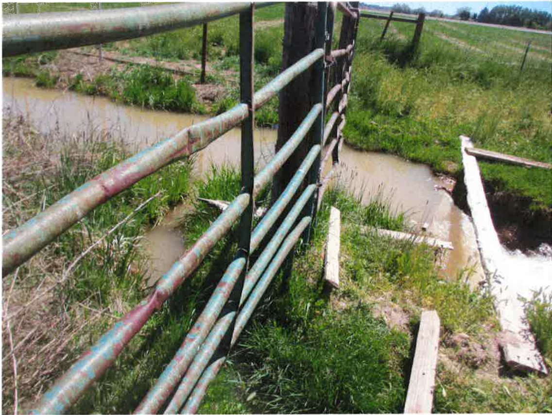
Point of Diversion - Ditch from Grouch Drain to regulating pond.
