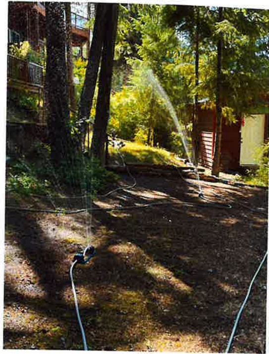
Multiple irrigation outlets on property to distribute water over land.
