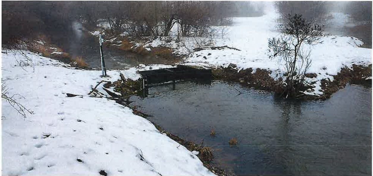
Figure 2: Weir on Mannon Ditch (has telemetry, but sensor had been removed by Watermaster)
