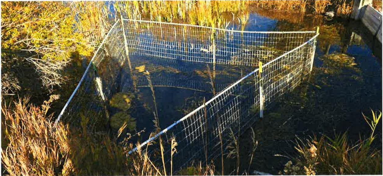
Figure 1: "Beaver Deceiver" at POD into culvert
