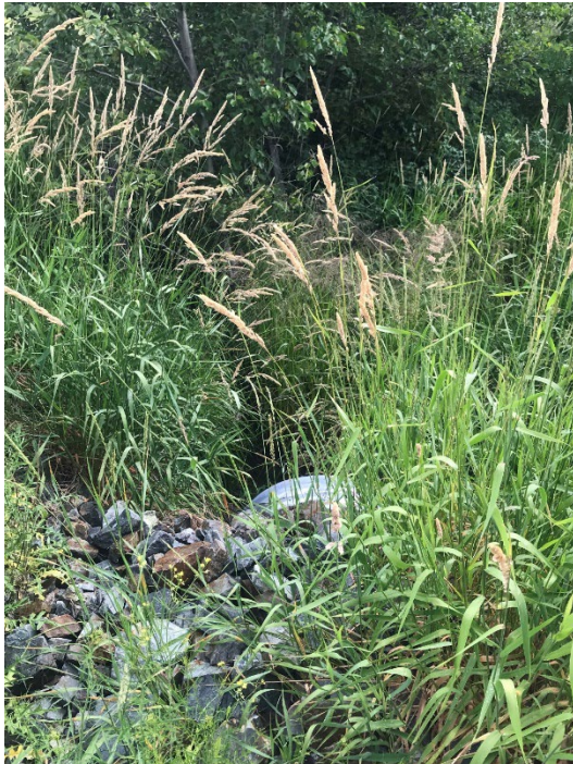
Culvert upstream across the road from the pump
