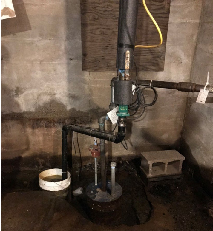
The well for the store and apartment is in the basement.
