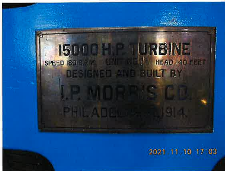
Photo 3. Turbine plaque typical of the three units.
