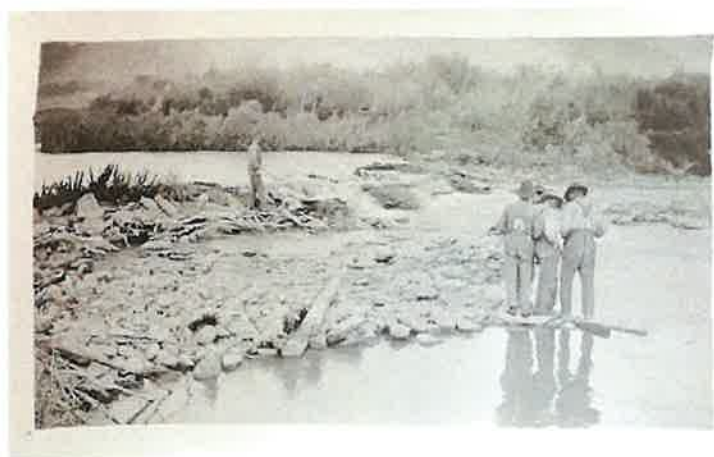
Figure 1. Historical photo of Wardboro Dam.
