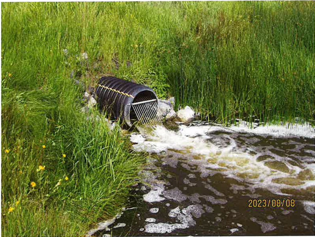
Photo 6. Outlet structure of large reservoir, looking upstream toward south berm.
