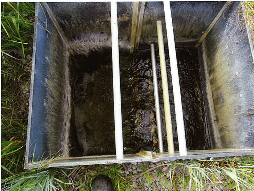
Photo 7. Outlet structure box at south berm.
