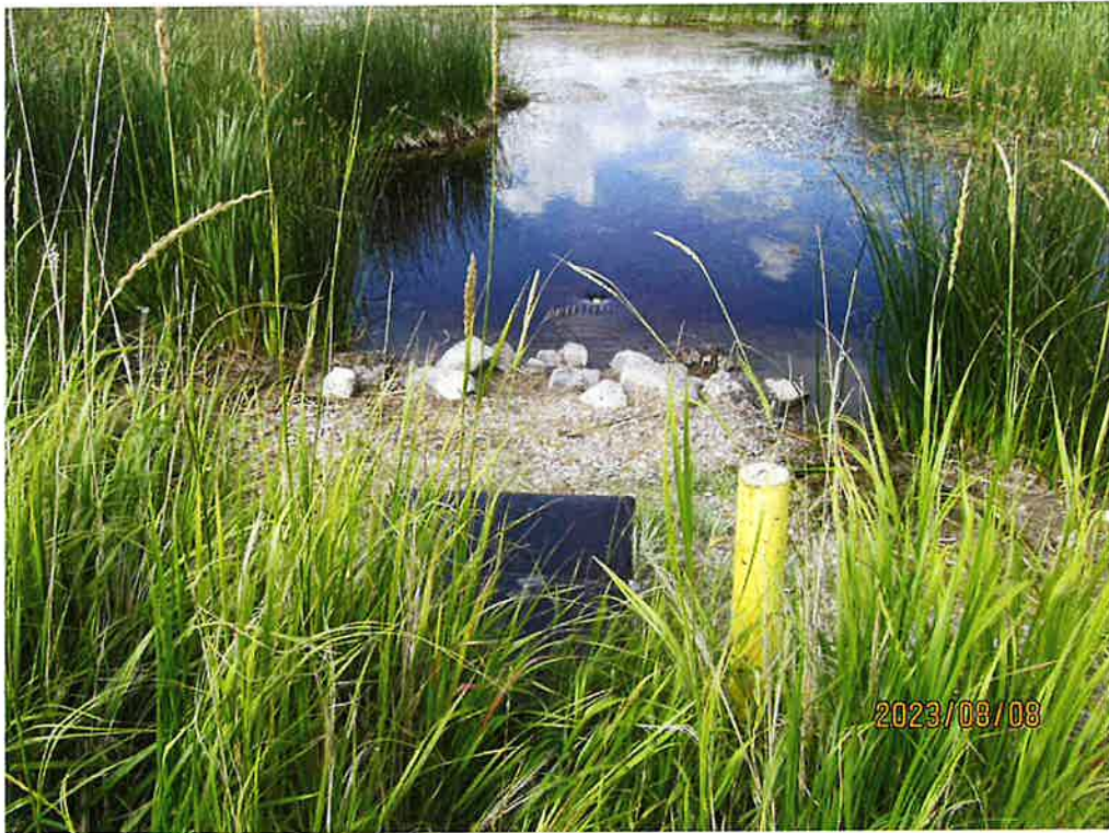
Photo 4. Inlet Structure to large reservoir, looking upstream.
