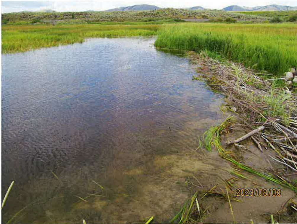
Photo 1. Looking East at the rock gabion structure of north berm, beaver activity also visible. Gabion structure is mostly submerged at this location. Water flows over the top.
