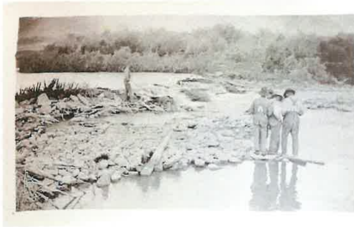
Figure 1. Historical photo of Wardboro Dam.
