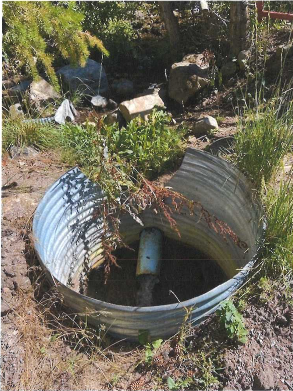
Diversion from Unnamed Stream
