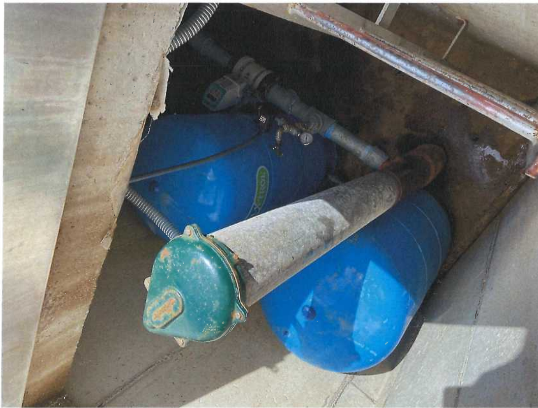
Well head in concrete vault.
