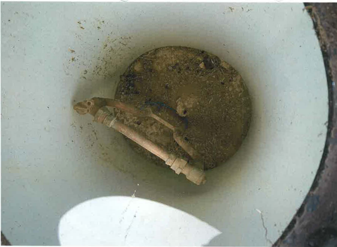
Fig. 9 – All lots that aren't developed yet have been stubbed in. View looking into a stub/meter.
