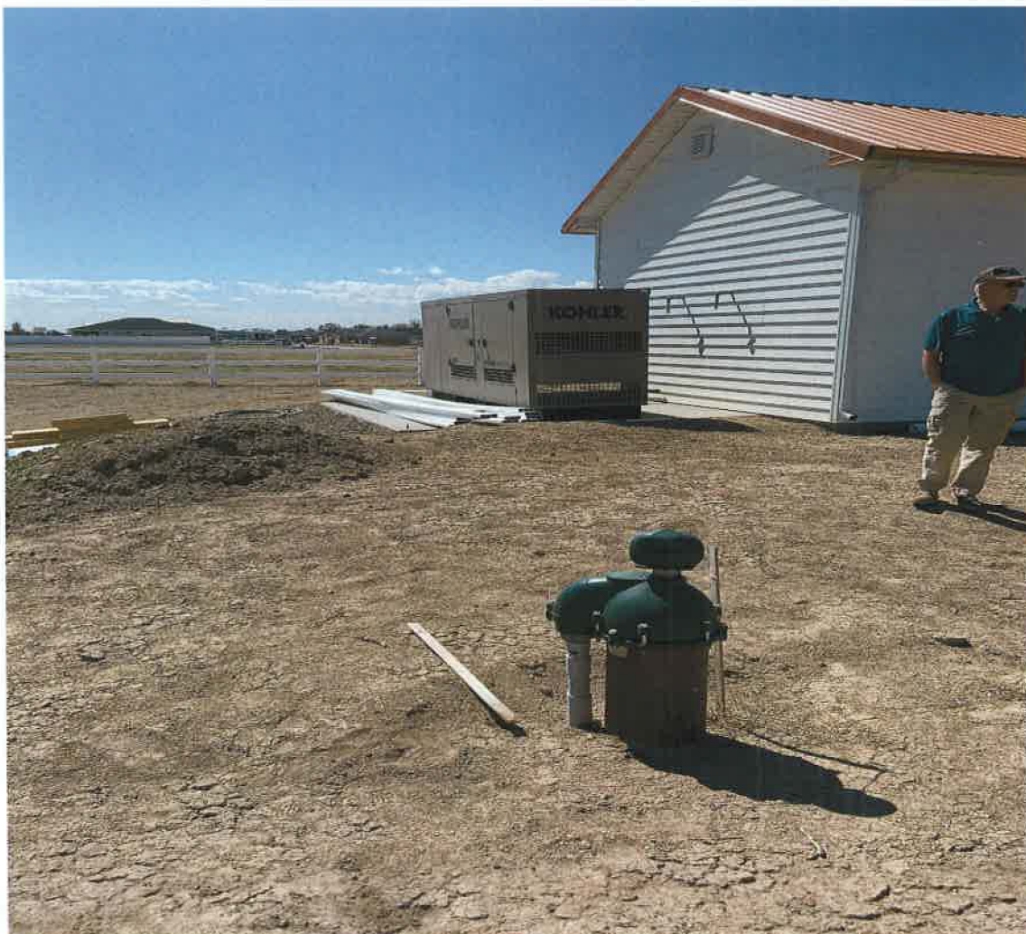
Fig. 2 – View of Well Tag ID D0078773 with pump house in the background.
