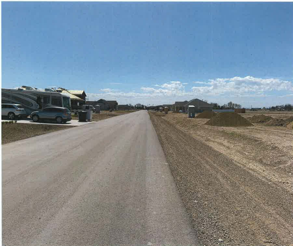
Fig. 12 – View looking south with block 1 to the left (east) and block 2 to the right (west). Lots are in different stages of development.
