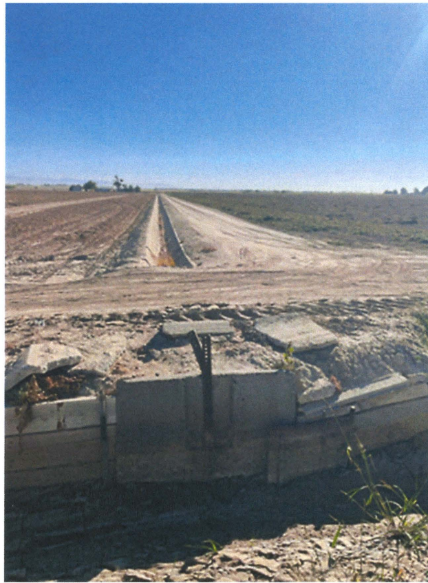
Figure 9 Photo of irrigation diversion and ditch that delivers water to a 40-acre section of the place of use. Photo was taken facing West.
