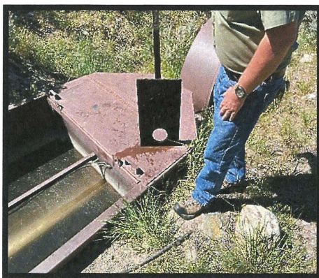
Photos 4 & 5 (left to right respectively) - 4. Orifice slip panel removed. 5. Overflow orifice is enclosed downstream of the fish screen. Rotary screen drum drive line between the water wheel and drive chain in the right of the image.
