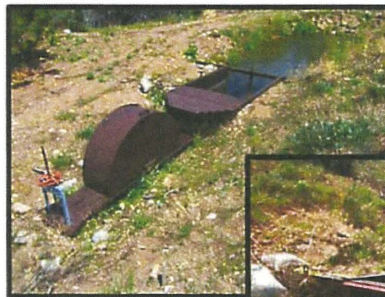
Photo 6- 10" PVC fish bypass on the left with overflow on the right, returning flow to Canyon Creek.
