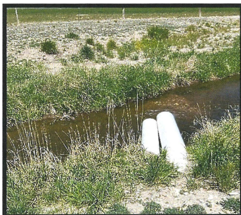
Photo 3- (left) Orifice slip panel removed from the right side of the enclosure. Photo 4- (Right) 10" PVC bypass pipe with the 10" PVC overflow pipe on the right of it returning flow to Eighteen Mile Creek.
