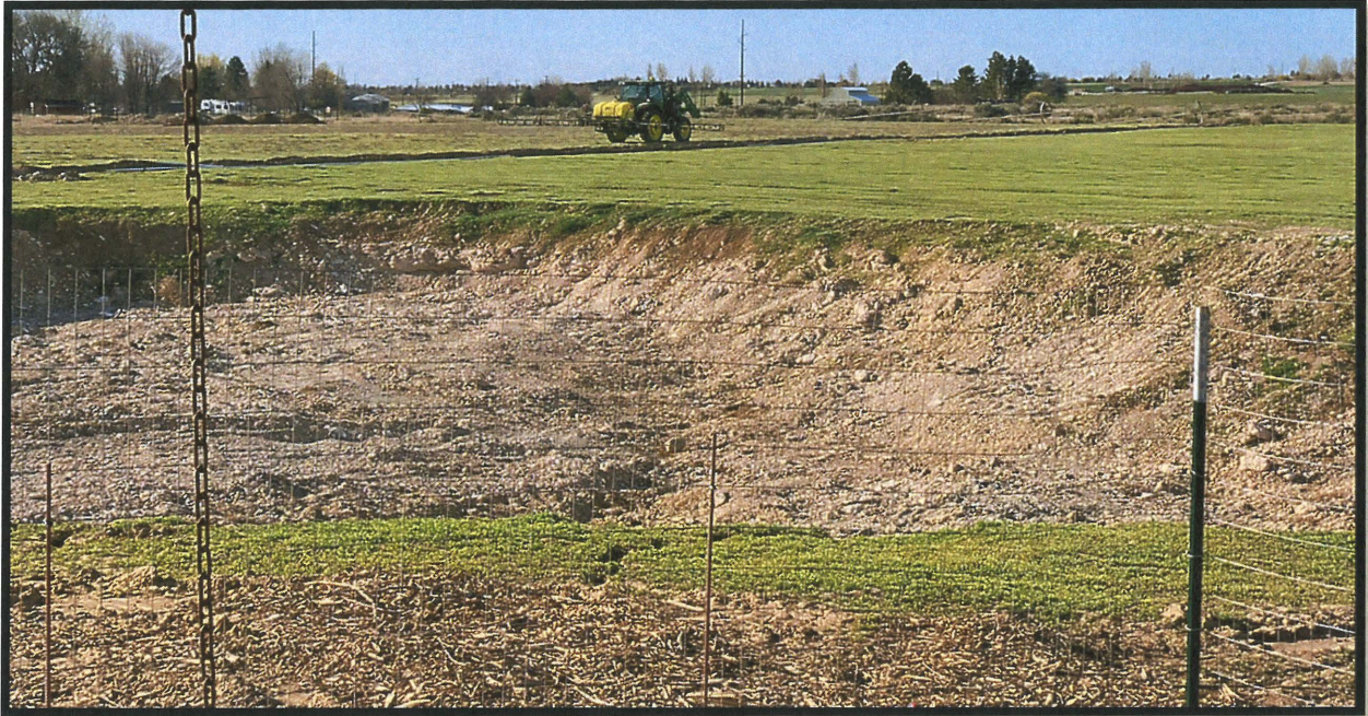
Photo 1 -c.2020—Taken by permit holder from back porch facing northwest. The pond under excavation.
