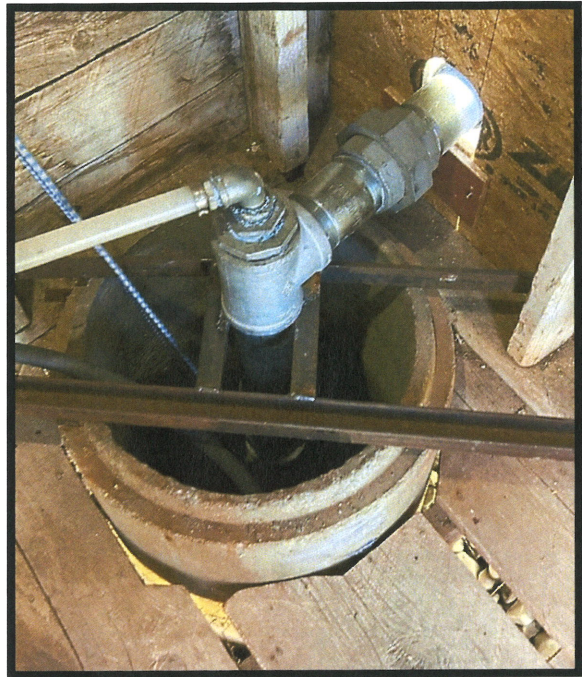
Photos 1 & 2- Left to right respectively. (1) Pump house facing northeast. (2) Drywell with 4" steel line exiting through the pump house wall. Photo 3-(lower left) Pressure tank. Photo 4-(lower right) Irripod as used in irrigated areas.
