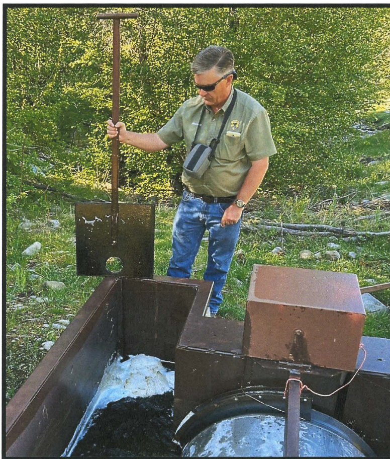
Photo 4- Orifice Slip panel removed by Mike Demick (IDFG escort). Centered approx. 2 ½ in above the bottom of the enclosure.
