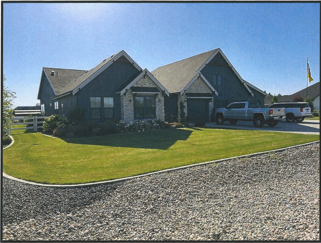
Photo 2- Standing at the northwest corner facing southeast irrigated beds surrounding the home and lawn along the north side of the home with the fire pit area in the background in the left center of the image.
