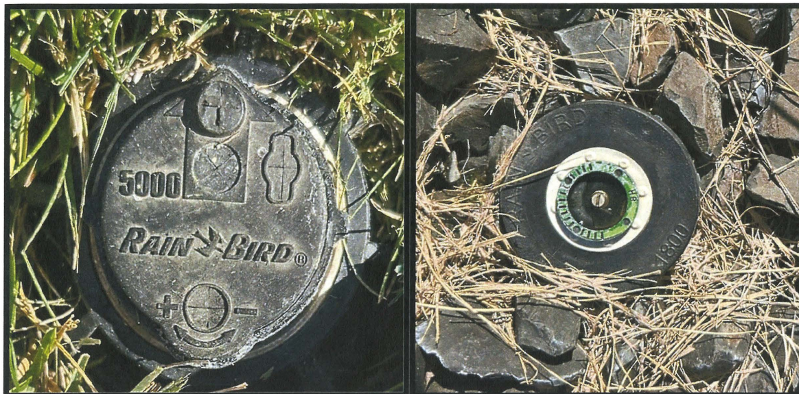
Photo 5 (Left)- Rain Bird 5000 series rotary sprinkler heads found throughout the larger zones in the POU. Photo 6 (Right)- Smaller Rainbird 1800 umbrella sprinkler head like those found in the landscaped beds of the POU.
