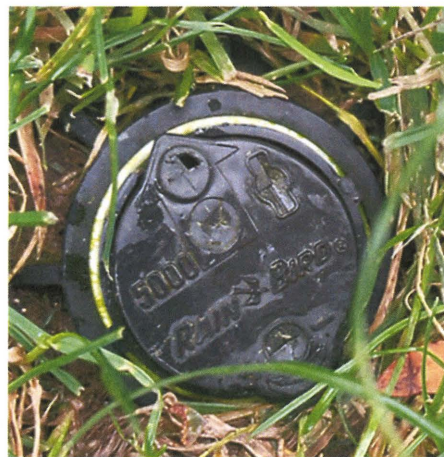
Figure 8 Rain Bird 5000 sprinkler head located within the irrigated area of property.
