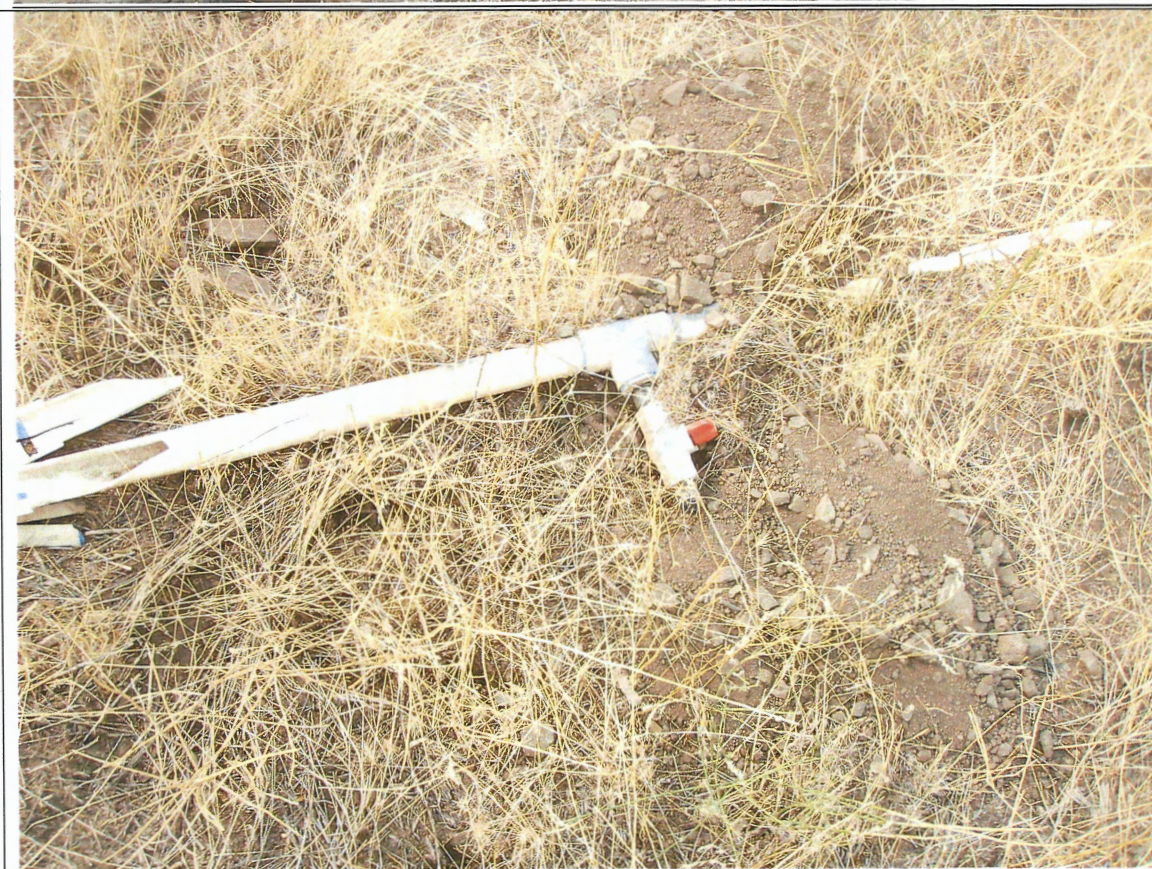
Figure 4. Remnants of 1 1/2 inch pipe and ball valves for irrigation which was initially developed for a small grape vineyard but was later abandoned.
