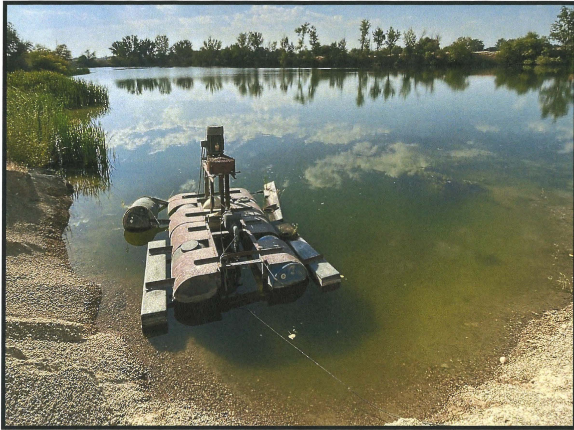
Photo 1 (above)- Facing southeast from the northwest bank of the storage pond. Pontoon pump station with 25Hp pump.
