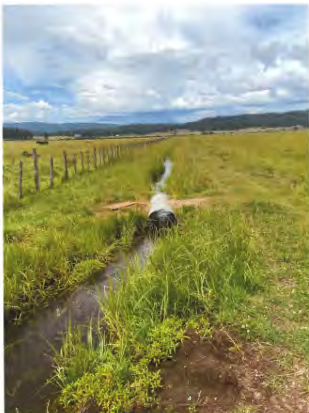
Fig. 8 – Wasterwater ditch conveyance parallel to the south of the POU. View looking W.
