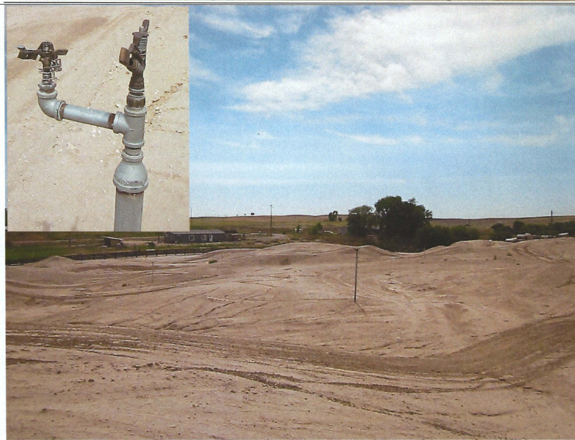
Figure 10. There are 68 fixed sprinkler sets mounted on vertical stand pipes with a 5 gpm discharge that are use for dust abatement on motocross tracks and a BMX track.
