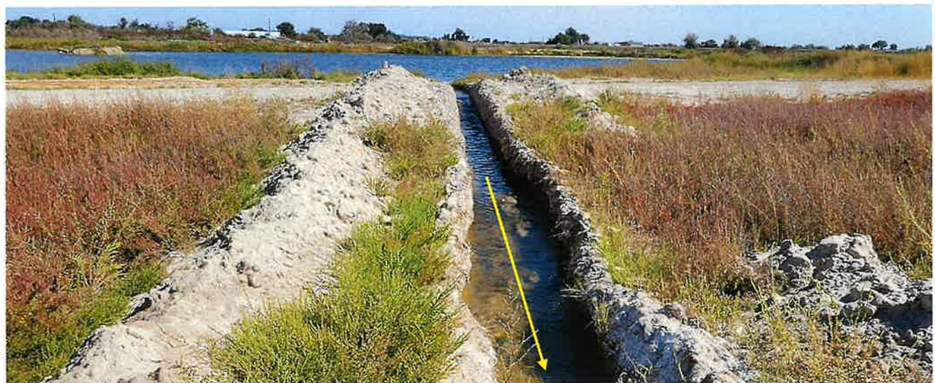
Photo 3. Image of the channel between the two ponds. Water is flowing from the east pond towards the west pond. The owner indicated that a buried pipe would connect the two ponds in the future.
