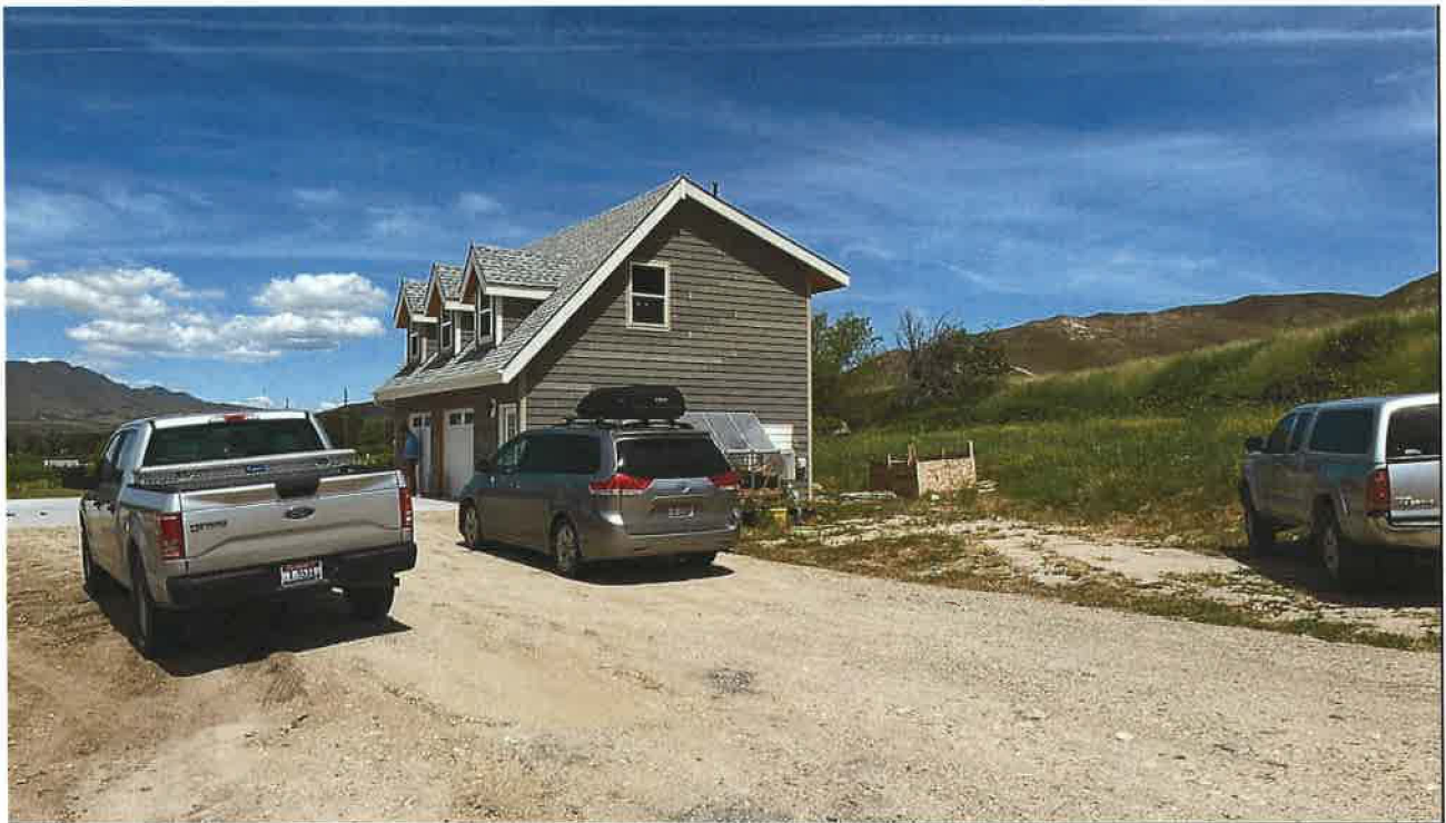
Fig. 4 –Detached garage with loft outbuilding.
