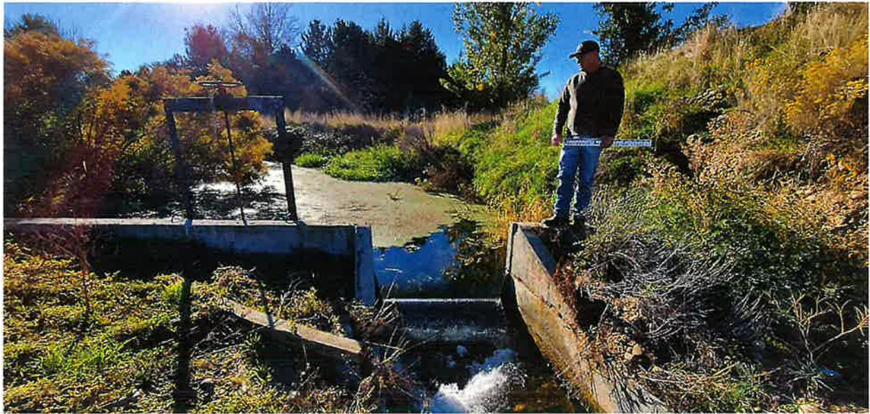
Figure 1: Doyle Fackler, Cipoletti Weir & Headgate
