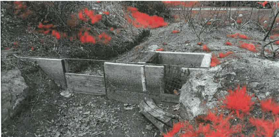
Split weir structure.
