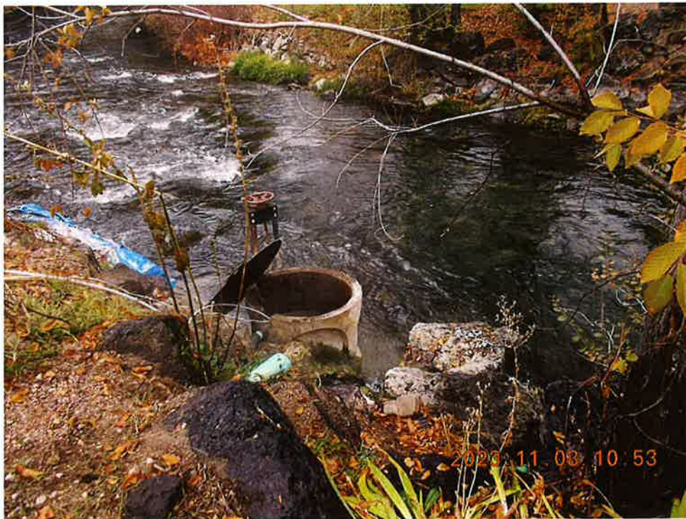
Photograph 2. Concrete geothermal spring box with metal cover removed, adjacent to the Portneuf River, viewing northwest.
