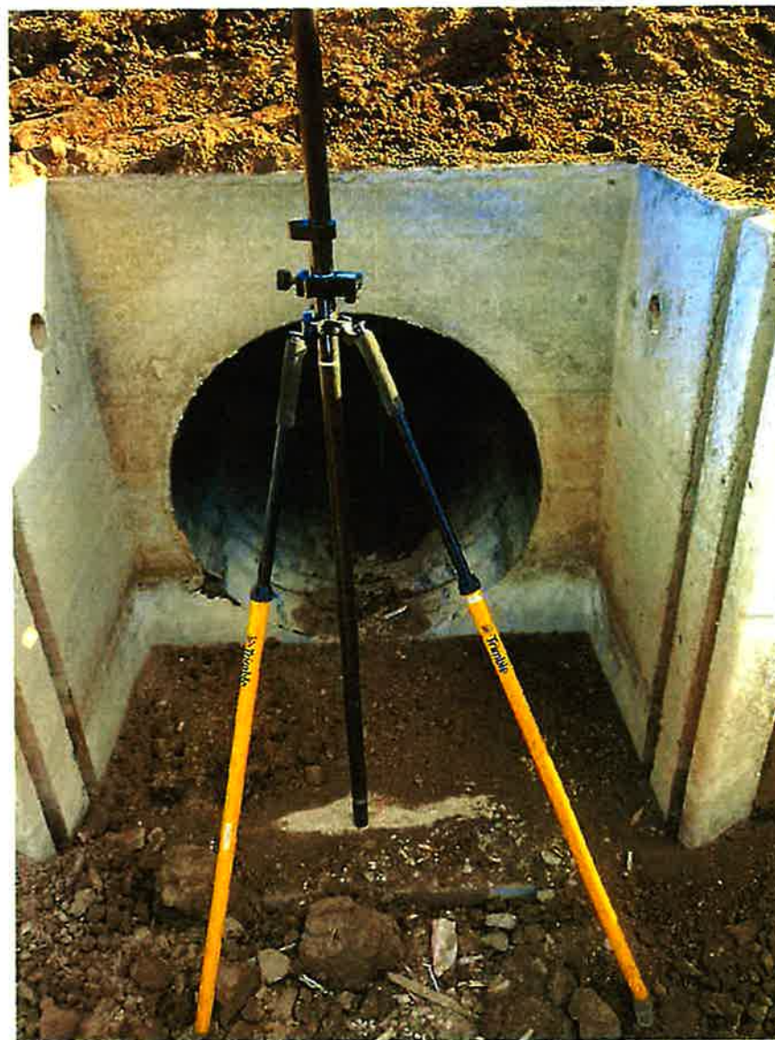
Photo 3. Internal view of 4-ft wide flashboard riser after installation. (Photo taken on 09/20/2022 by Steve Pilson, USFWS)
