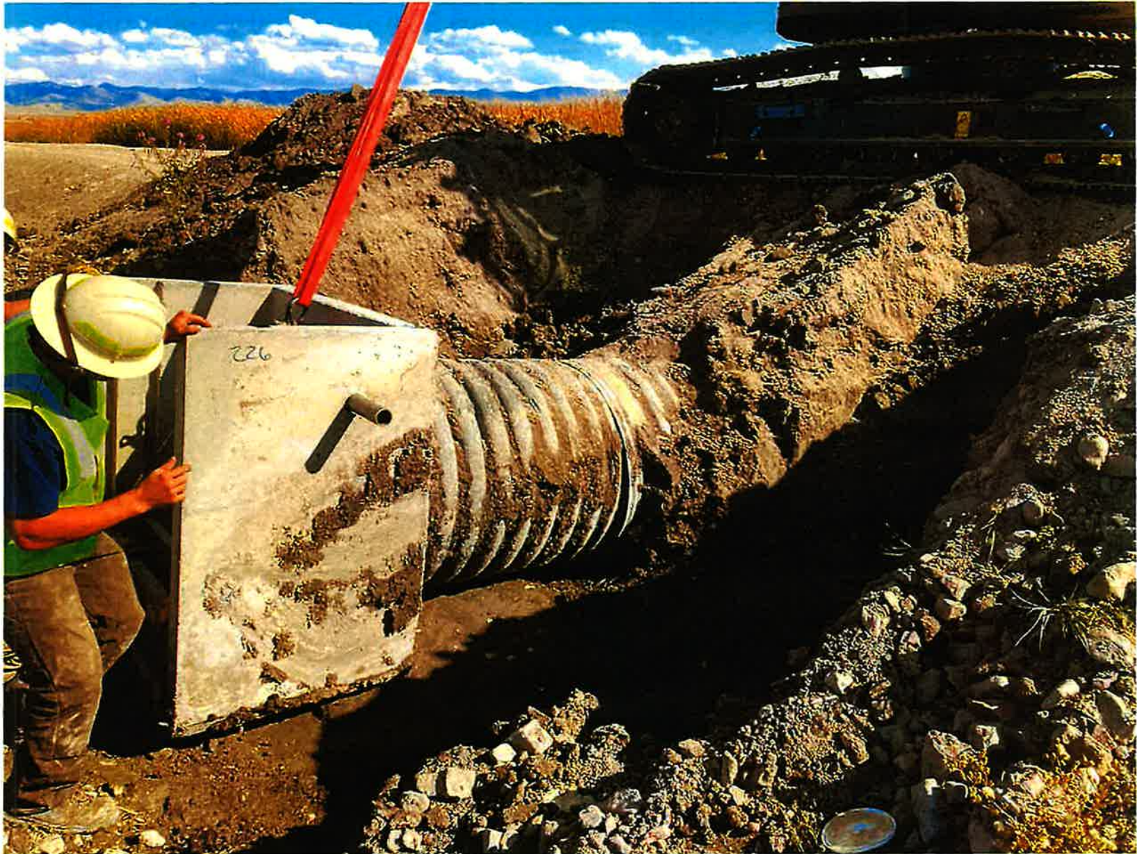
Photo 1. Installation of 4-ft wide concrete flashboard riser that functions as the water control structure at one of two points of diversion. This is the easternmost of the two points of diversion and is similar to the one located at the westernmost point of diversion. (Photo taken on 09/20/2022 by Steve Pilson, USFWS)
