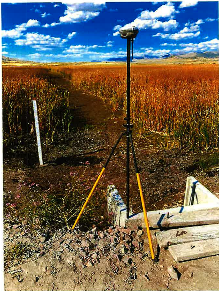
Photo 2. After installation of the 4 ft-wide concrete flashboard riser that functions as the water control structure at the eastern point of diversion. (Photo taken on 09/20/2022 by Steve Pilson, USFWS)
