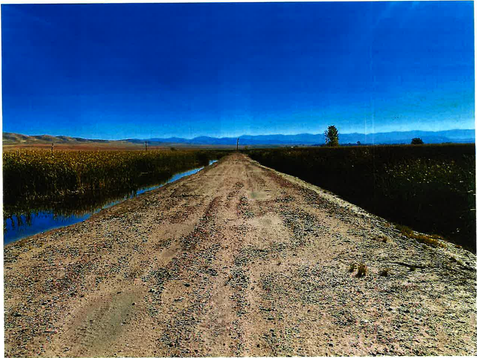
Photo 6. View looking east from the eastern point of diversion from the road atop the 4.5 high, 550-ft long dike that functions as the dam that stores water in the place of use. (Photo taken on 9/25/23 by Jeremy Jirak, USFWS)
