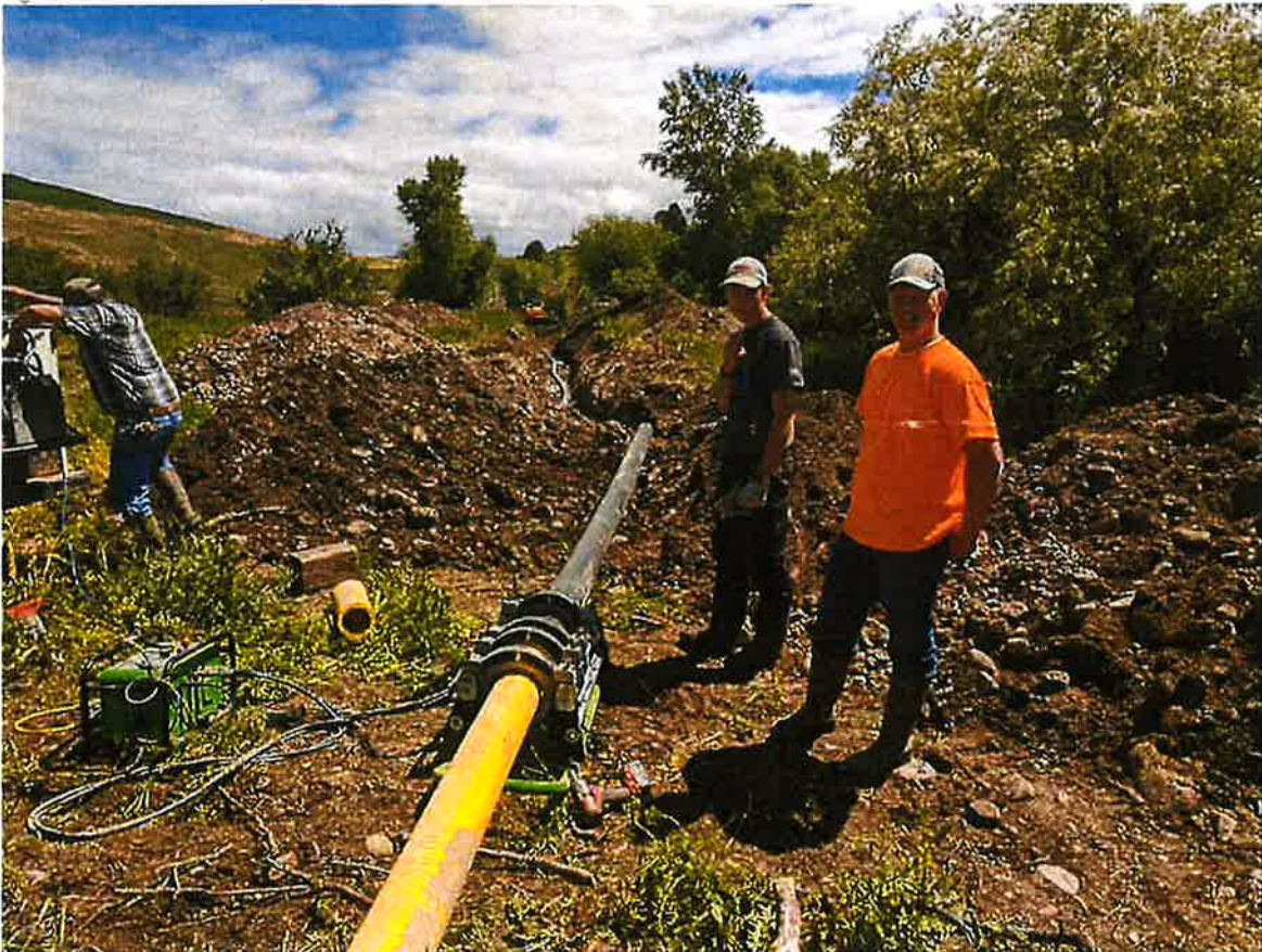
Figure 2 Hygee Fish Pond 6" HDPE June 18, 2020
