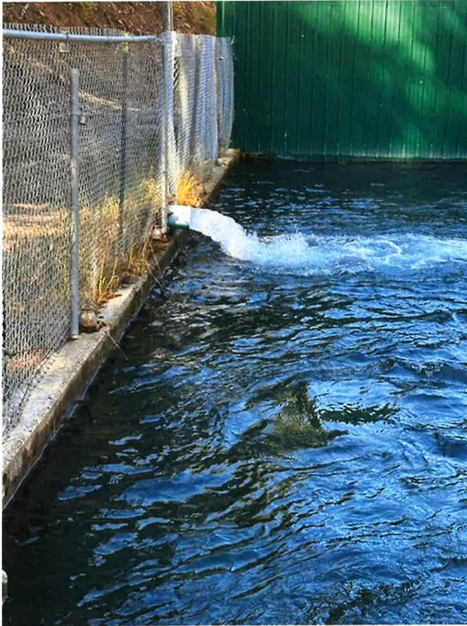
Stilling Pool at Pipeline Intake
