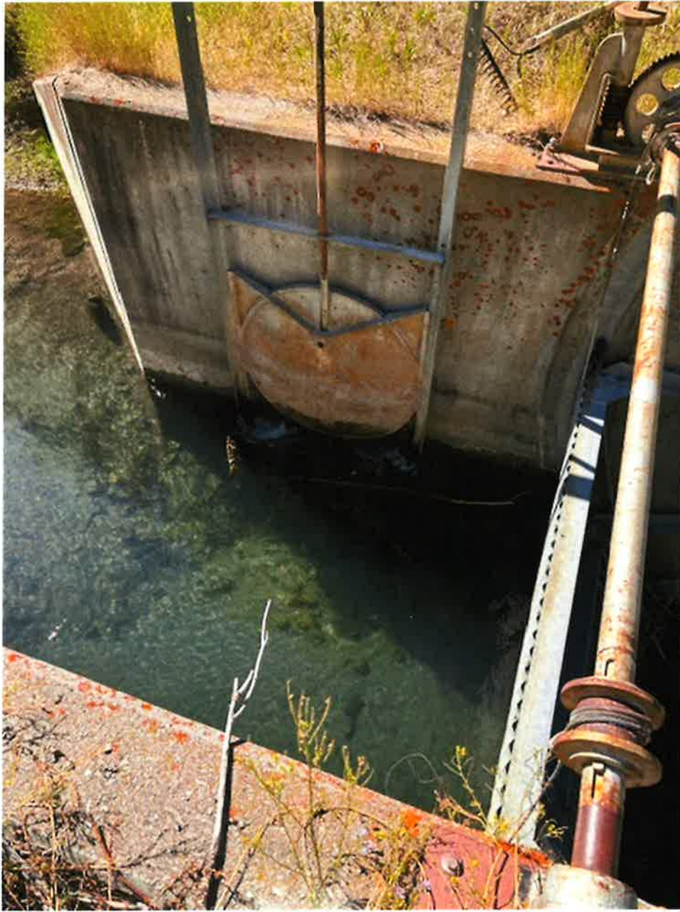
Georgetown Irrigation Company Diversion on Georgetown Creek Company diverting full flow of creek.
