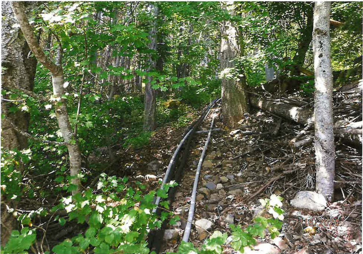
CONVEYANCE PIPELINE ROUTES UP STEEP GRADE APPROXIMATELY 340-FT ELEVATION GAIN TO STORAGE TANKS
