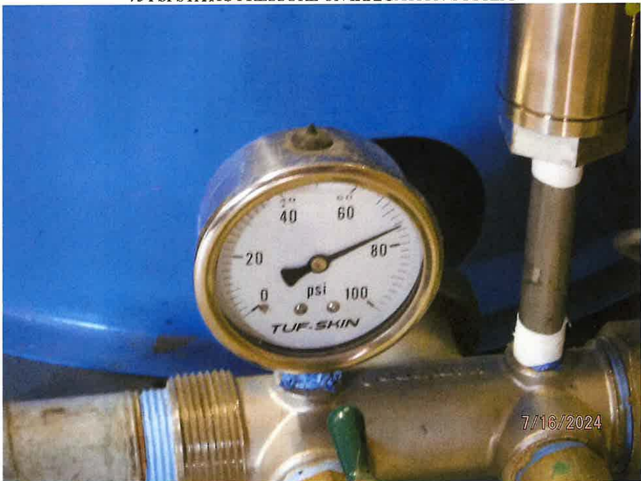
75 PSI STATIC PRESSURE ON IRRIGATION SYSTEM
