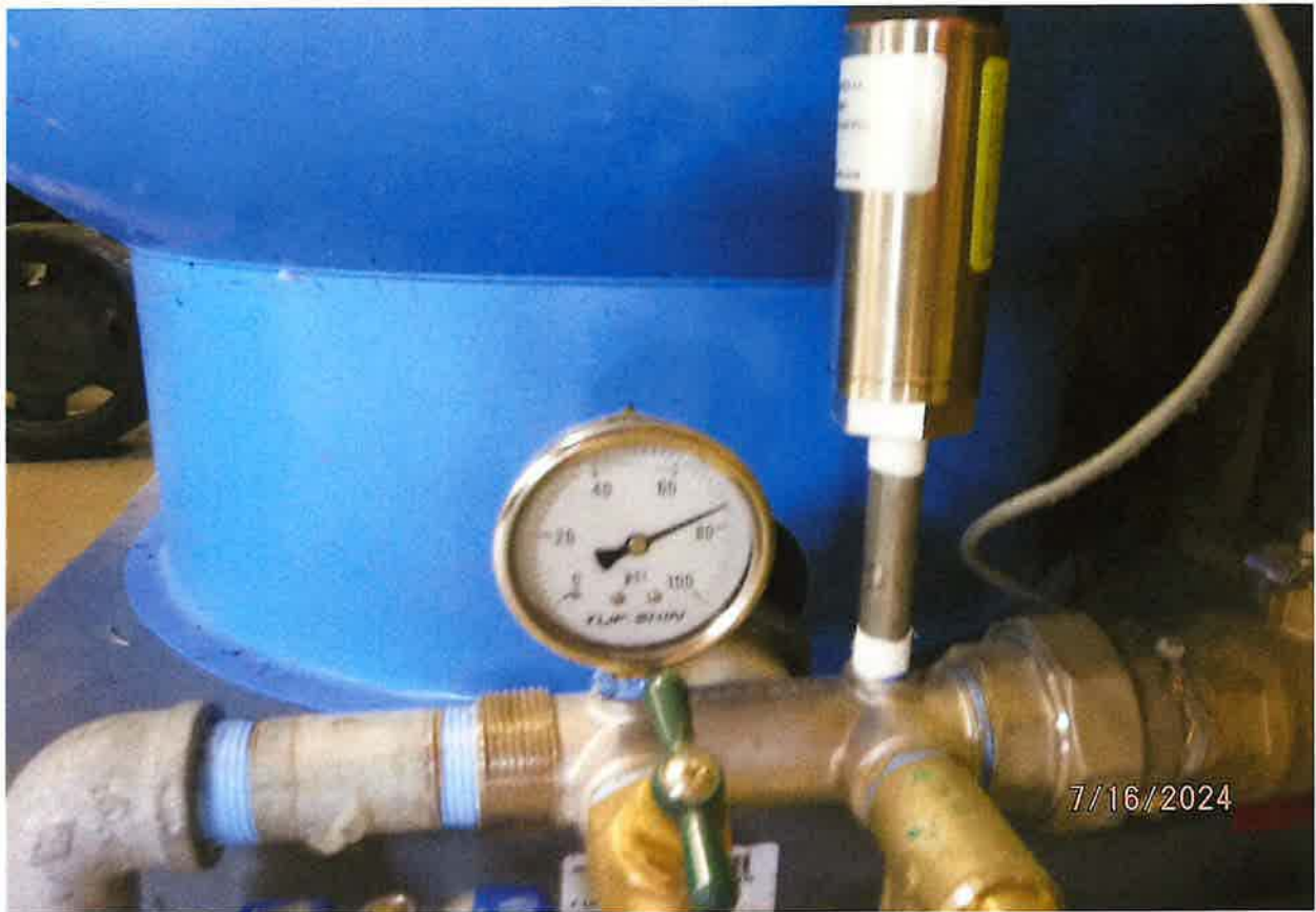
75 PSI STATIC PRESSURE ON IRRIGATION SYSTEM
