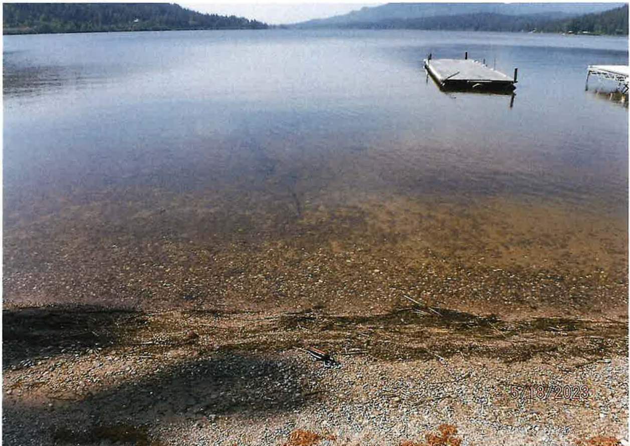
POD – SCREENED FOOT VALVE IN LAKE WITH POLY PIPE TO CENTERFUGAL PUMP
