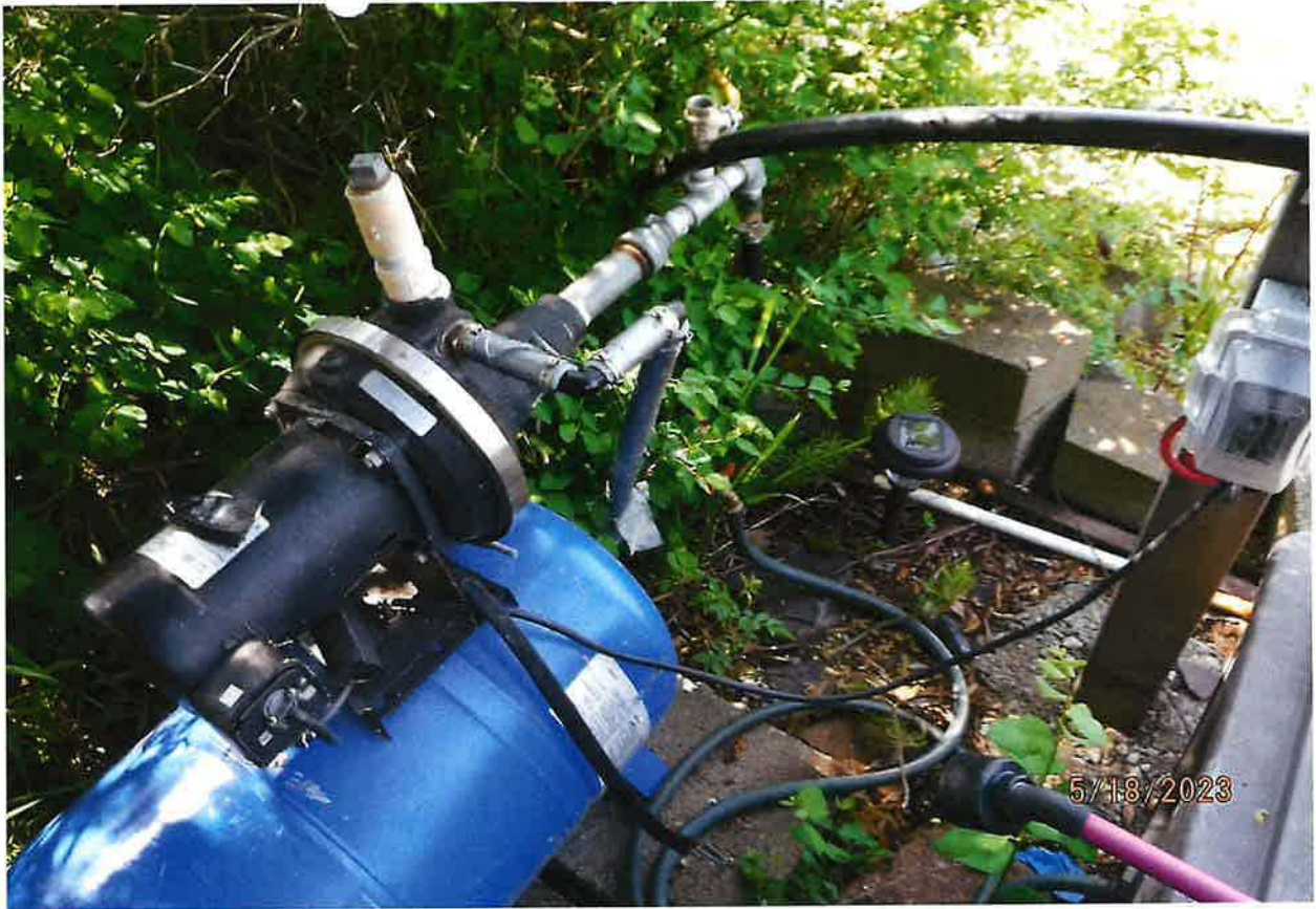
SEARS 1/2 HP PUMP & PRESSURE POT
