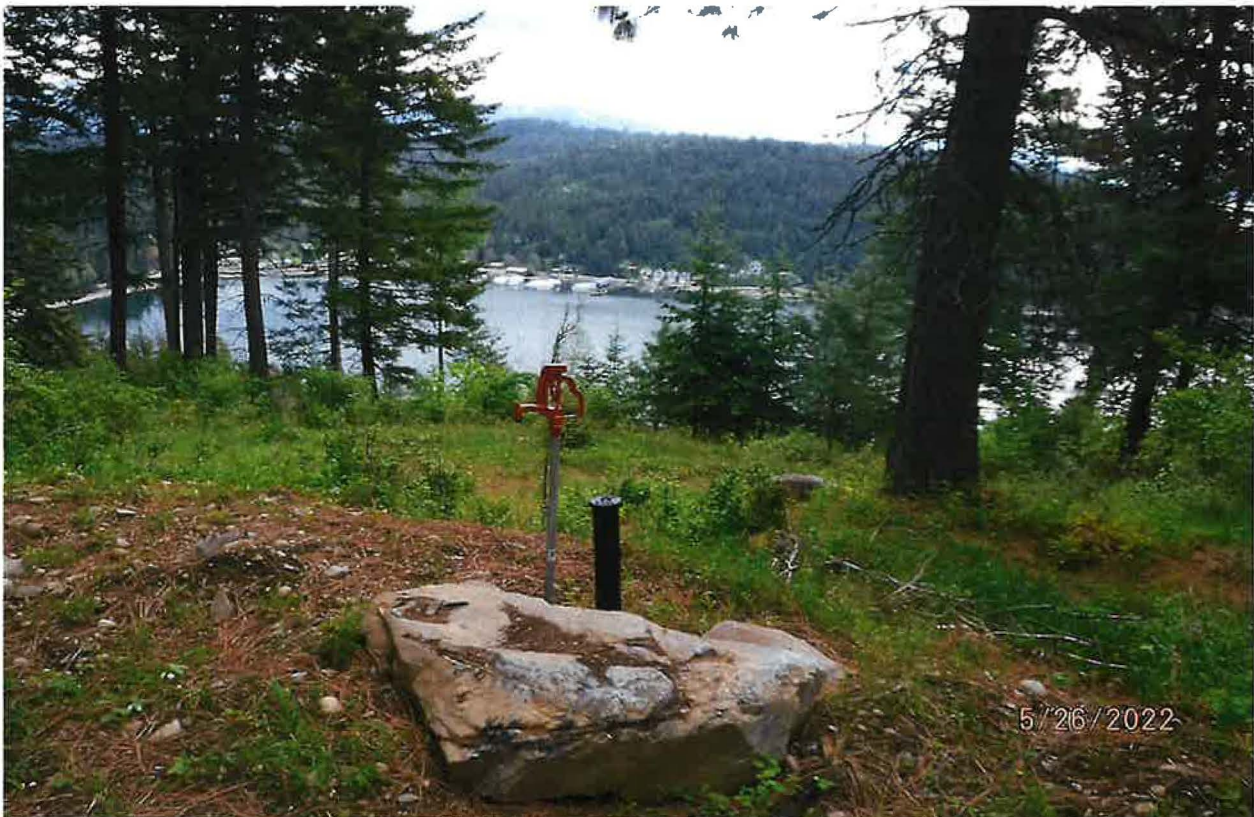
DOMESTIC POU – STUB-IN - LOT 11, GARFIELD VILLAS REPLAT LOT 1 SUBDIVISION. RP023520000110A
