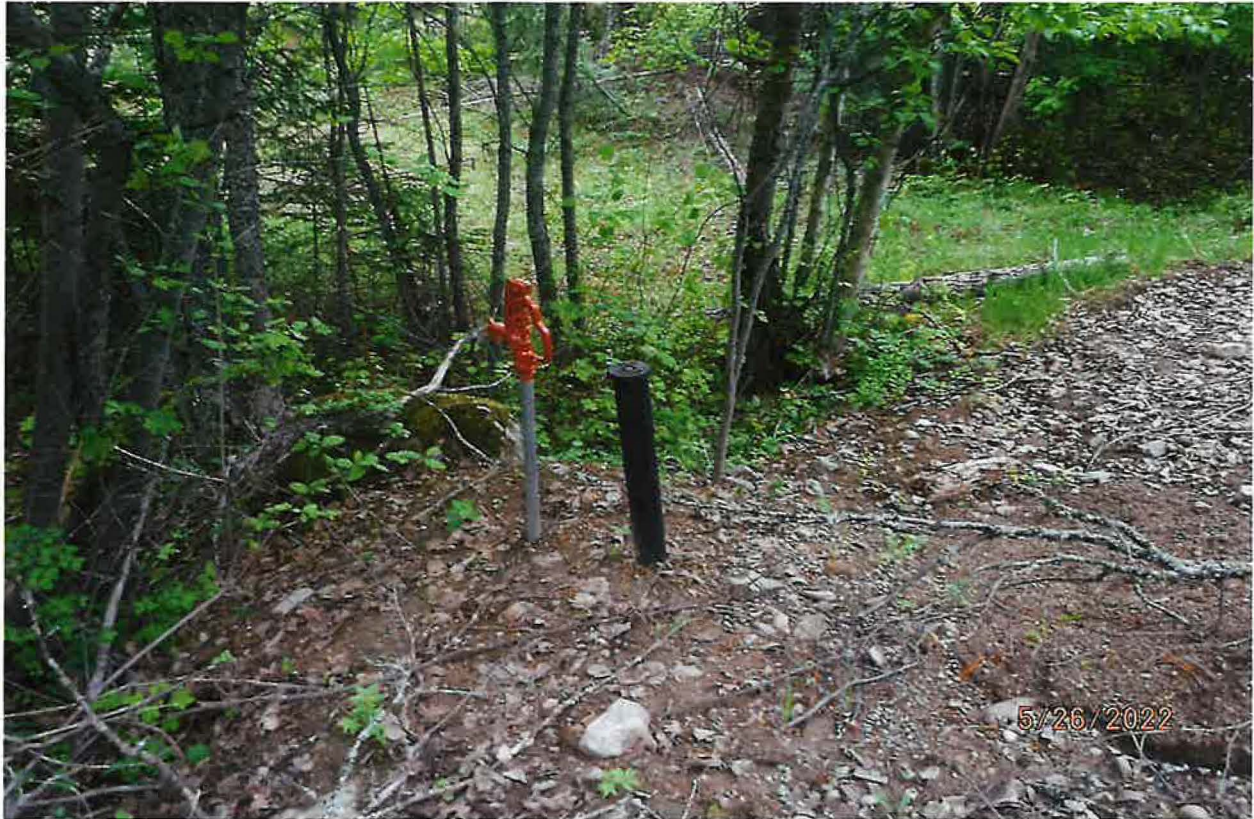
DOMESTIC POU – STUB-IN - LOT 8, GARFIELD VILLAS REPLAT LOT 1 SUBDIVISION. RP023520000080A
